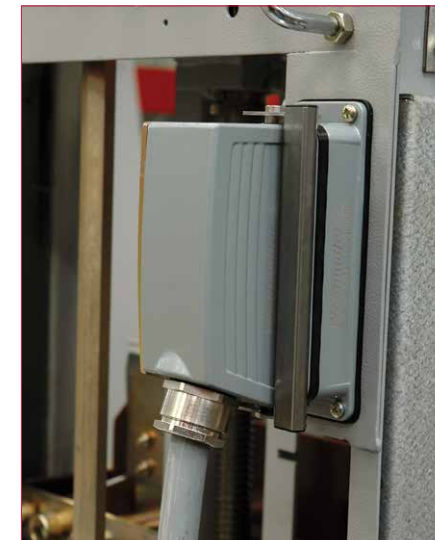
24 way plug and socket for secondary isolation
